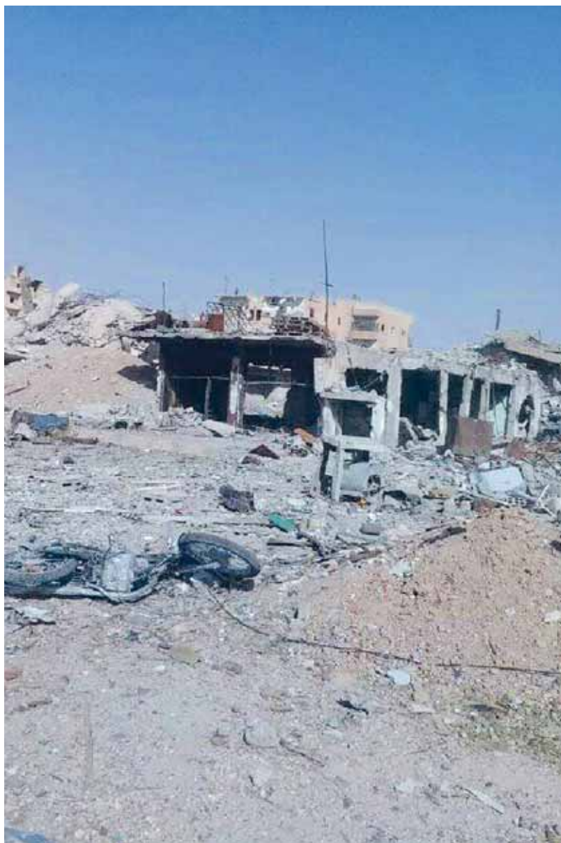
The house of Aziza al-Sharif Ibrahim, 70, the city of Raqqa, Raqqa governorate, destroyed in July 2017 by an American coalition air strike. Photograph: Aziza al-Sharif Ibrahim
