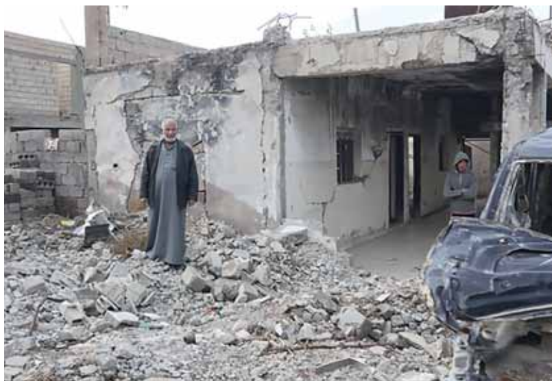
A house destroyed by US-led coalition strikes in the town of Hatlah, Deir ez-Zor governorate. Photograph: volunteers of the Foundation for the Study of Democracy
