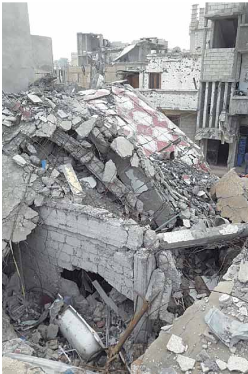
Photo: the house of Abta Al-Hasan Mustafa (58 years old), the city of Raqqa, Raqqa province, destroyed in July 2017 by a US-led coalition air strike. Photo courtesy of Abta Al-Hasan Mustafa
