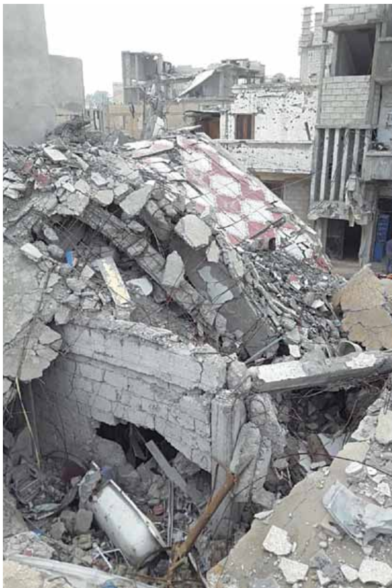
House of Abta Al-Hasan Mustafa (58), destroyed by an air strike of the US coalition in July 2017, city of Raqqa, Raqqa governorate. Photograph: Abta Al-Hasan Mustafa
